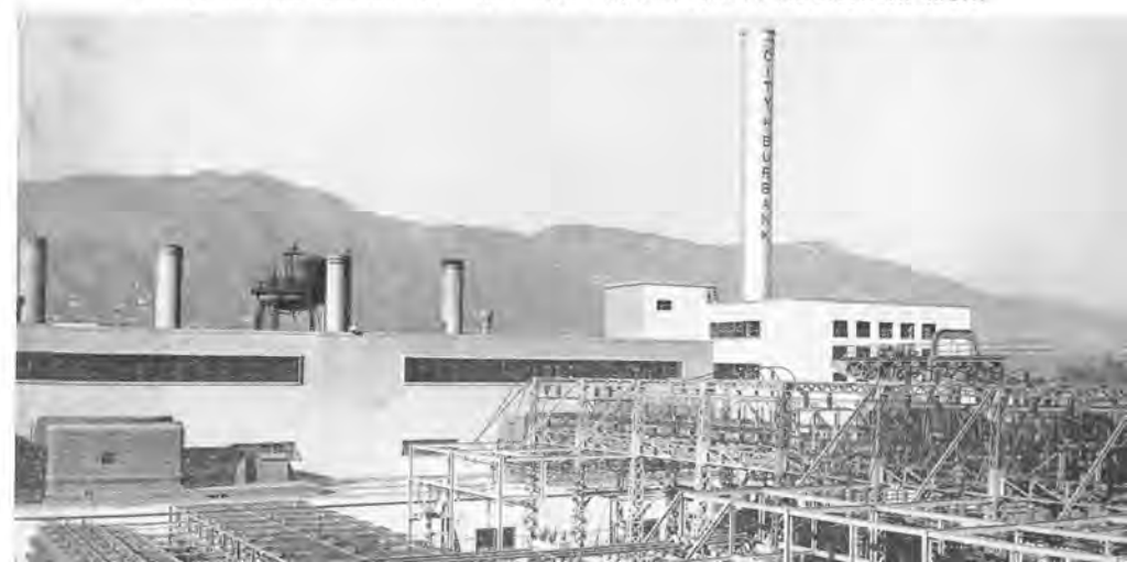
STEAM-ELECTRIC GENERATING PLANT—NEW 20,000 KILOWATT ADDITION AT RIGHT
