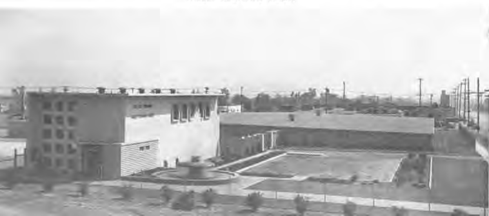
VALLEY PUMPING PLANT
