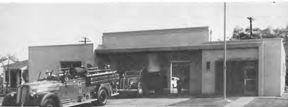
NEW FIRE STATION NO. 5
