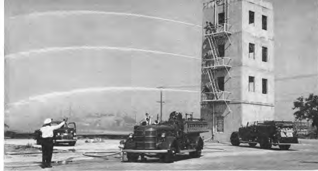
NEW FIRE DEPARTMENT TRAINING TOWER
