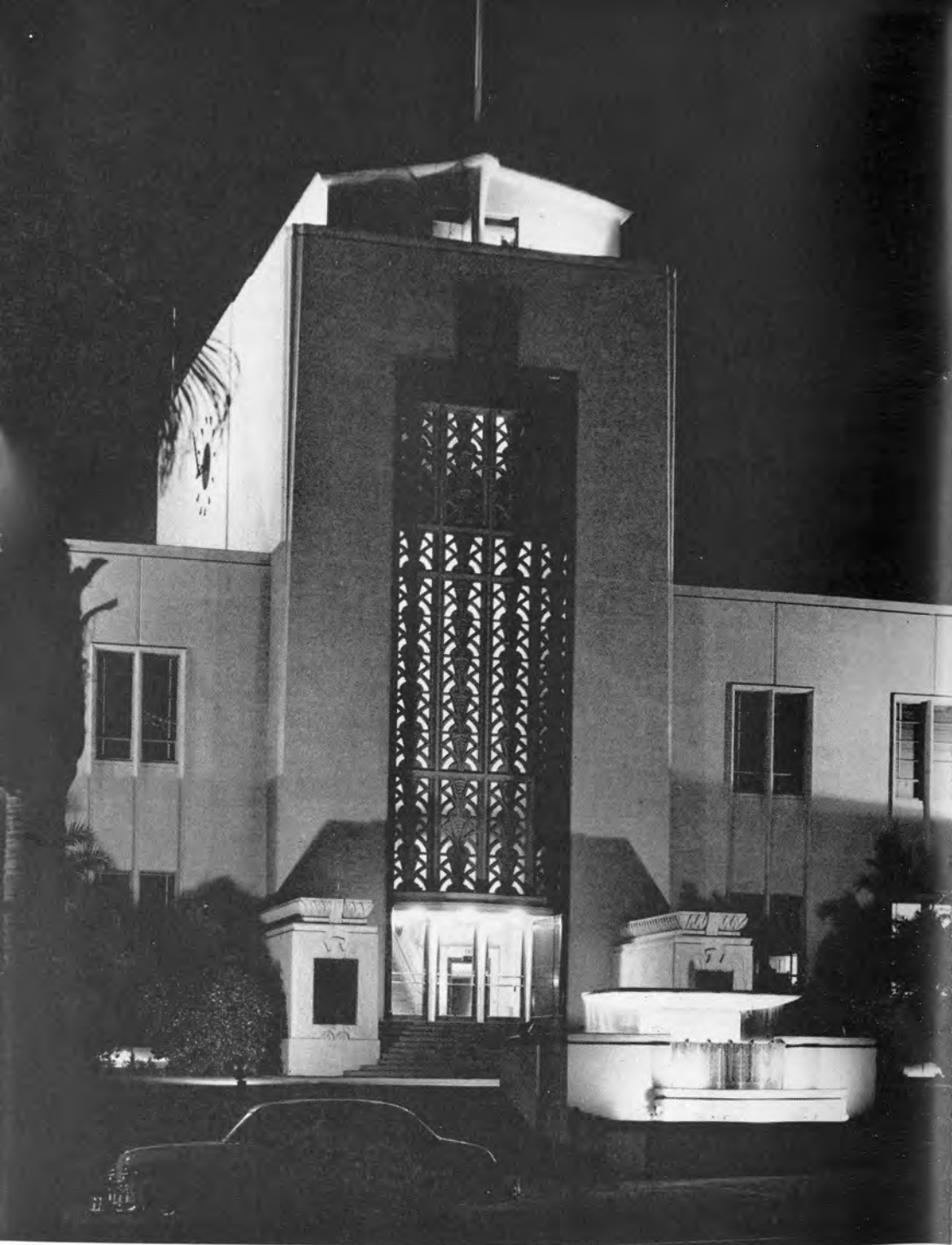
The City Hall — Main Entrance
