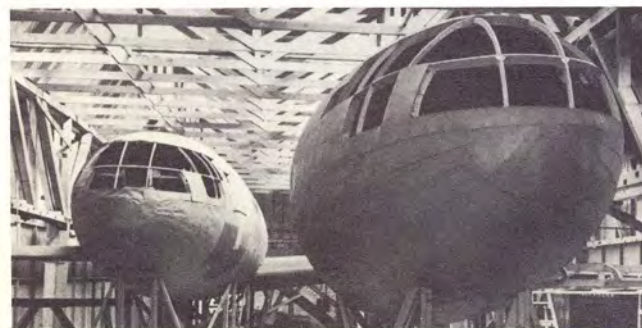
Excalibur A became first Constellation design. Several different windshield and cockpit layouts were evaluated.
