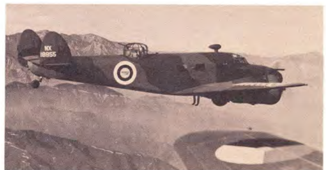
Lockheed offered Model 12 as three planes in one: for attack with bombs, nose guns, defensive gun turret; photography and observation; and speedy transport. Camouflaged plane above served Dutch in East Indies, aided evacuation during Japanese invasion. Left below, bombs on belly of Model 12. Right, window holes were for firing small arms.
