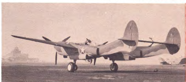
High tail P-38, above, failed to solve compressibility problem. Below, Lightning production rate hit 15 daily.
