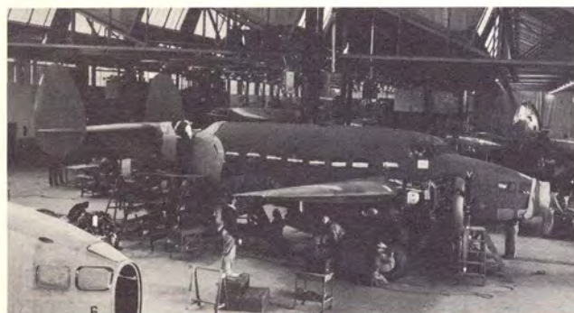
Hudson assembly, shown in early stage in February 1939, enabled Lockheed to pioneer mass production techniques.
